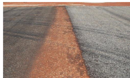
Sealtuff-Flex with grit added
